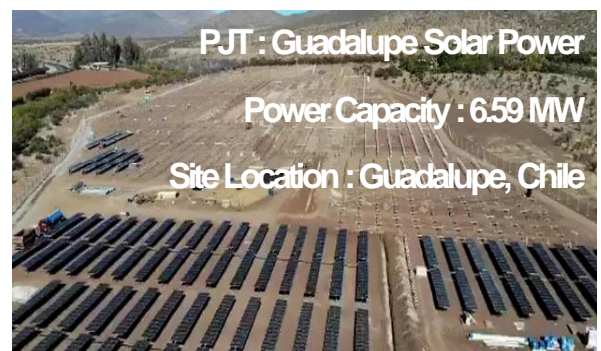
Modules of the Guadalupe Solar Power Plant Being Installed (28 June)
