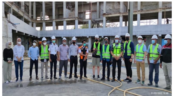
New Bus Terminal Construction Site in Samarinda City
